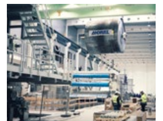
Lifting into the machine hall
