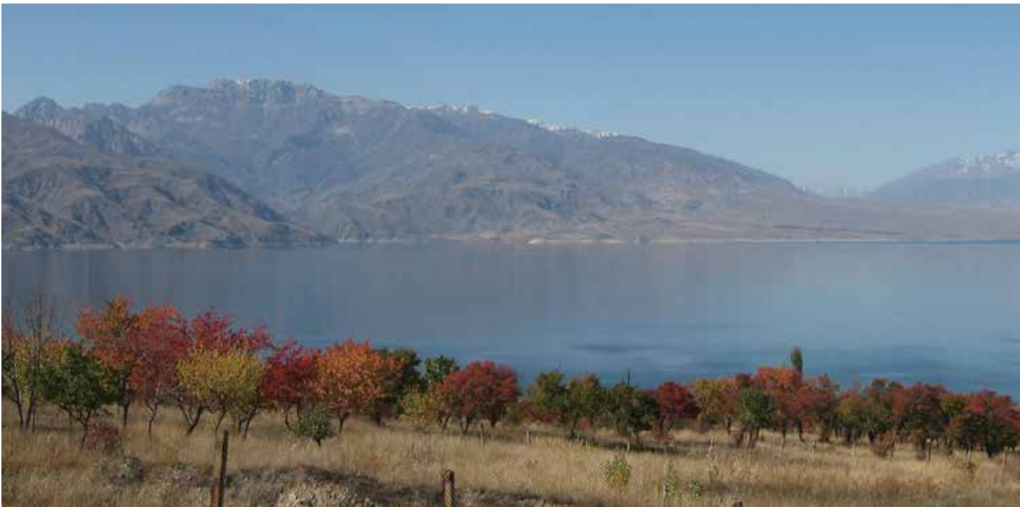
The reservoir at the 1,200 MW Toktogul hydro project on the Naryn River (Kyrgyzstan), which is currently undergoing rehabilitation and upgrade
