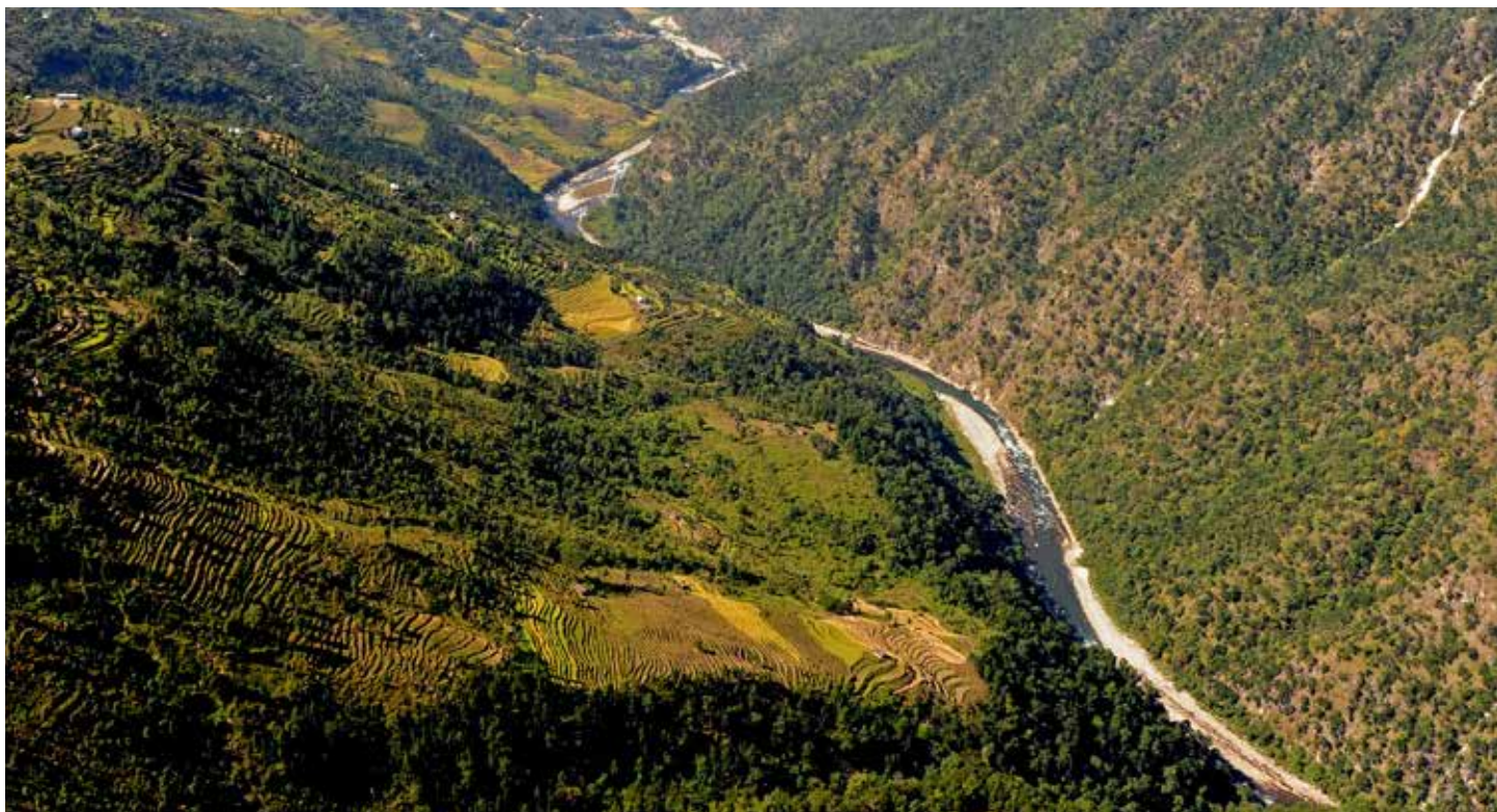
The site of the Kabela A hydropower project in Nepal, which undertook a protocol assessment in September 2014
