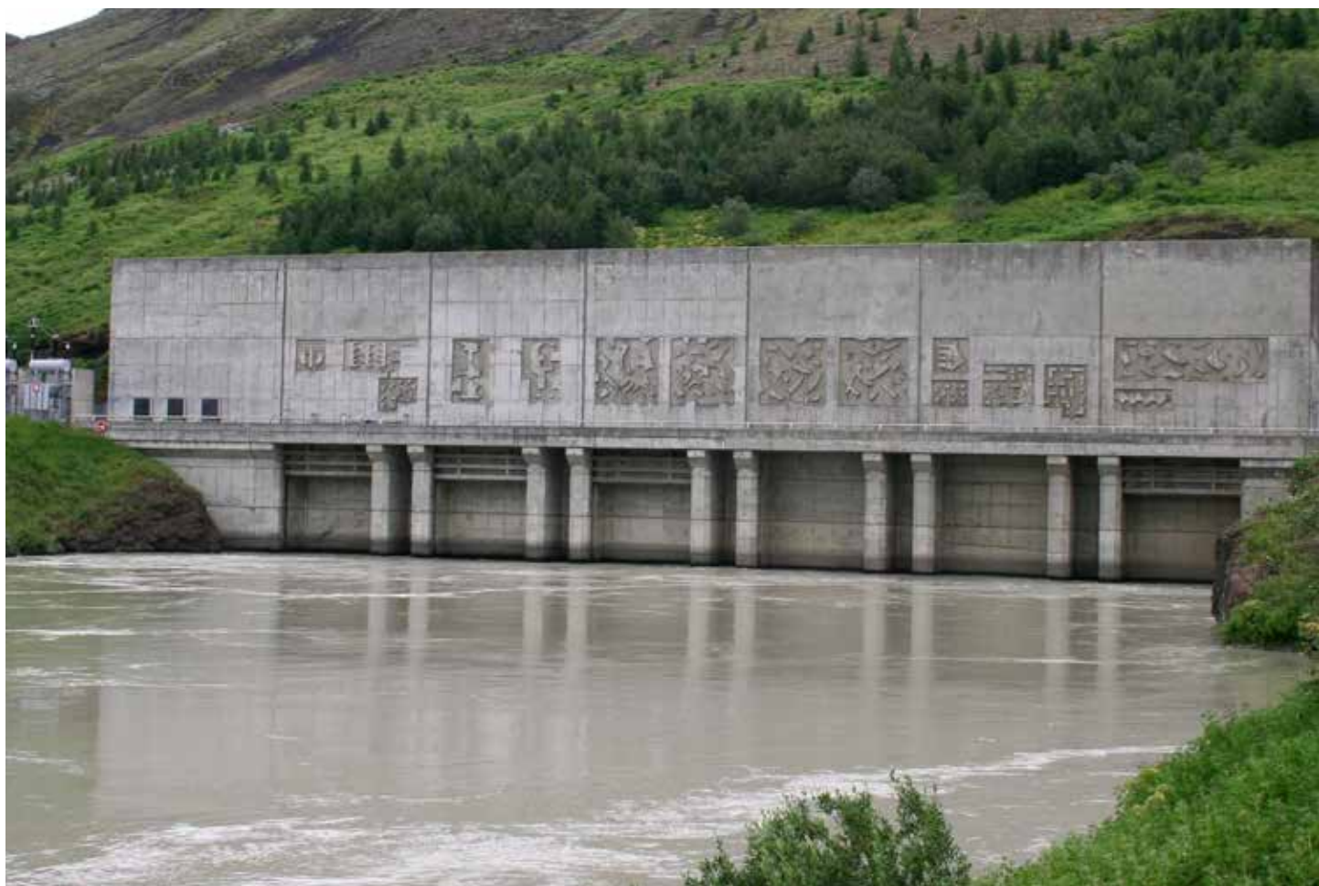
The Búrfell hydropower plant in Iceland, owned and operated by Landsvirkjun, is being expanded to cope with expected increases in flow rates
