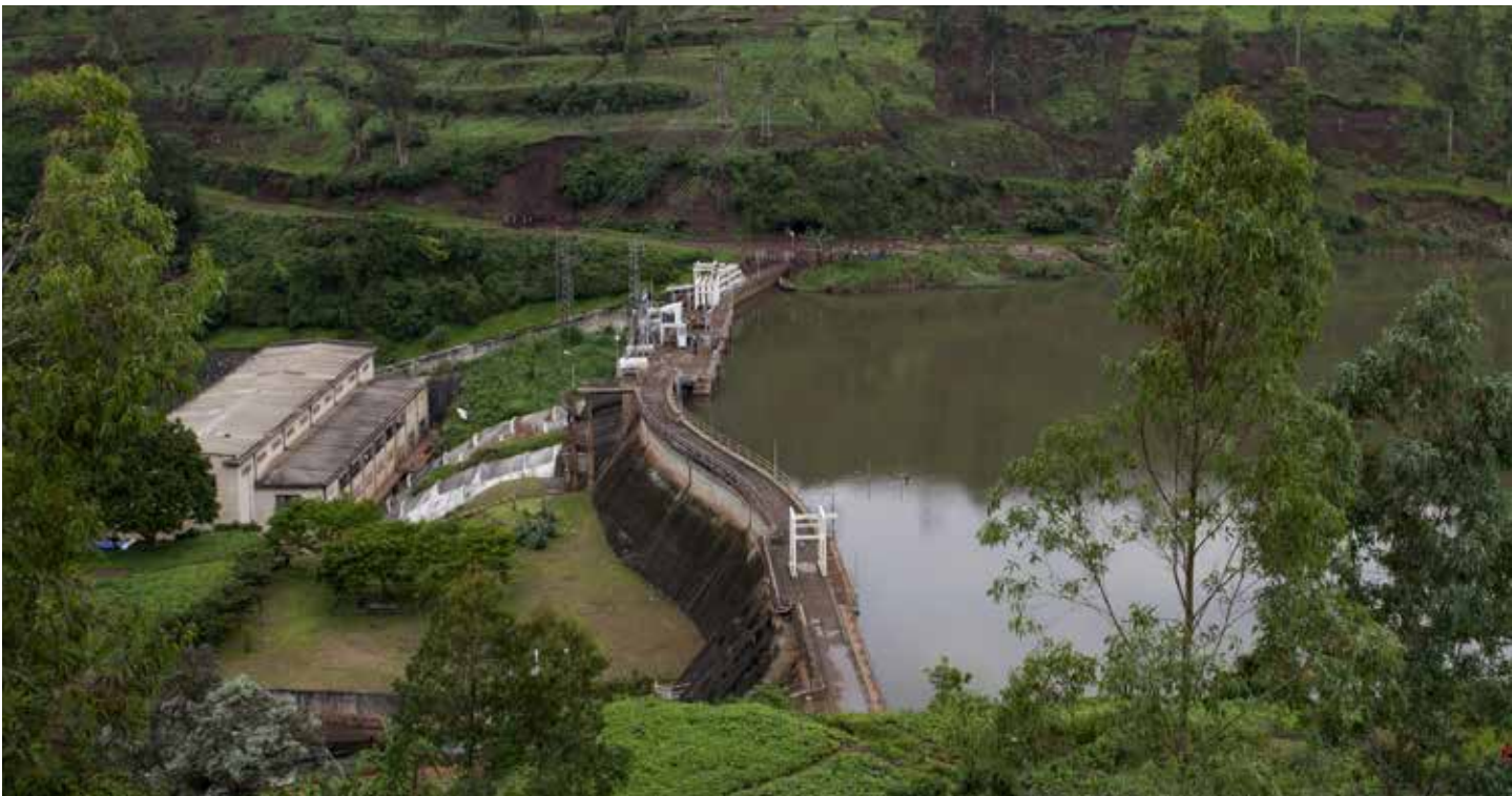
The Ruzizi I hydropower plant on the Ruzizi River, bordering Rwanda and DR Congo
